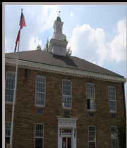
Pickett County Courthouse
