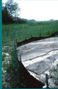
Silt Fences temporarily pond runoff and retain sediment on-site, often as perimeter control.
