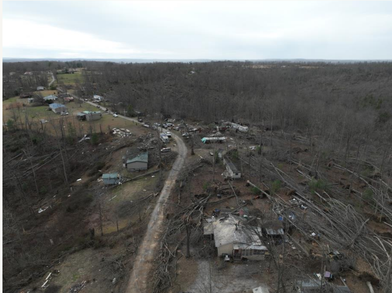
Weather events, washouts, debris, landslides, bridge approaches
