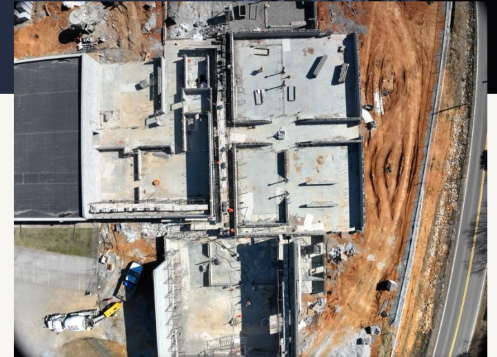
Progress records, staging areas, paving, guardrail corridors
