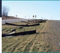
Silt Fences temporarily pond runoff and retain sediment on-site, often as perimeter control.
