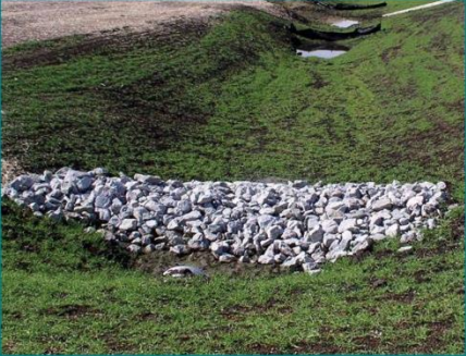
Rock Check Dams prevent gully erosion caused by concentrated flow.
